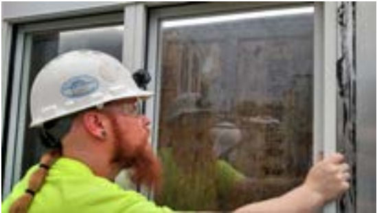
Field Service Member checking the seal on a sliding window
