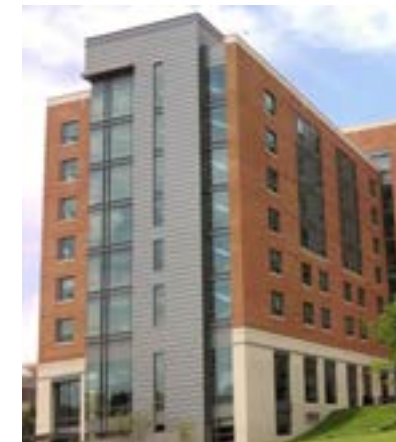
Prince Frederick in College Park, MD used a small Window Wall System to add a dramatic corner to the building.
